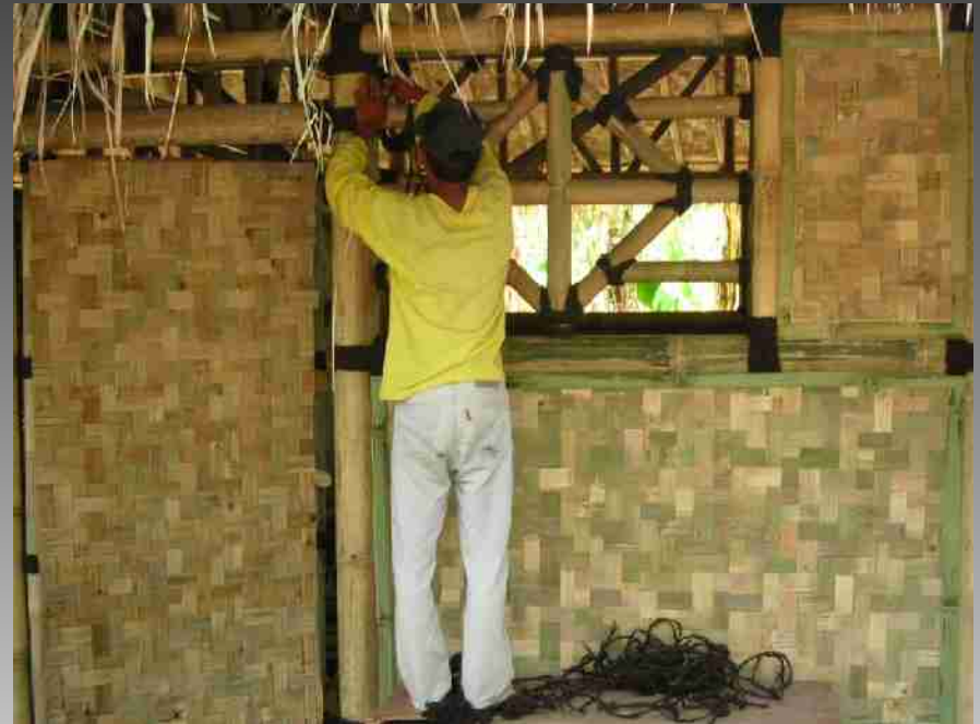
Constructing temporary schools using Bamboo, Indonesia
